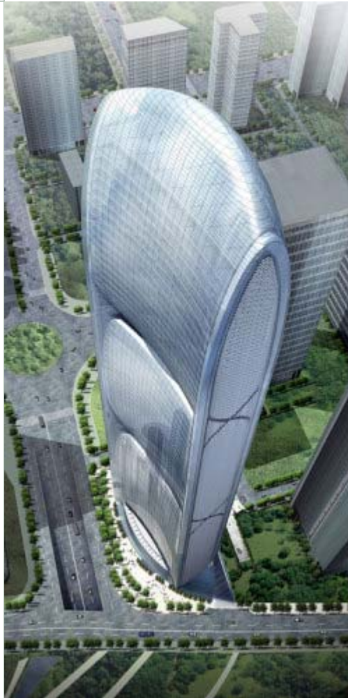
The Pearl River Tower will include four vertical-axis turbines located in penetrations through the face of the building.
